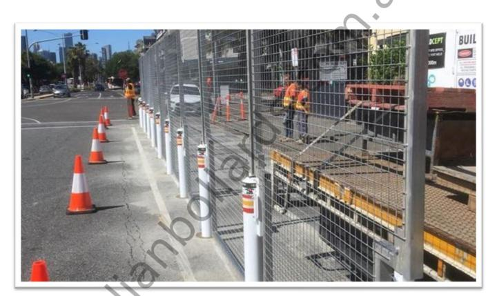
AB-EAB — Energy Absorbing Bollards with metal fence and AB-FD300-Solar powered flashing Amber LED on the head.
